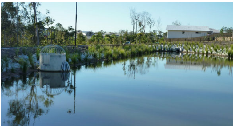
Fig. 1.5 A typical retention basin
