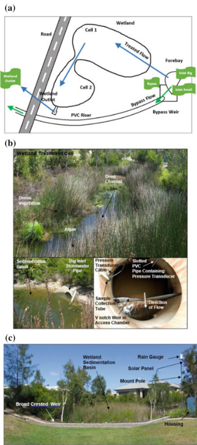
Fig. 2.6 The constructed wetlands. a Aerial view of the constructed wetland. b The constructed wetlands at the site. c The bypass weir
