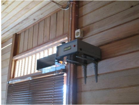
Fig. 3. Installation of smart shading device equipments.
