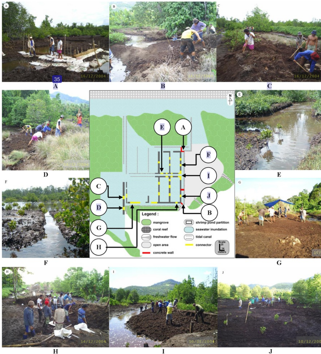
Figure 3. Physical changes to restore the hydrological condition
