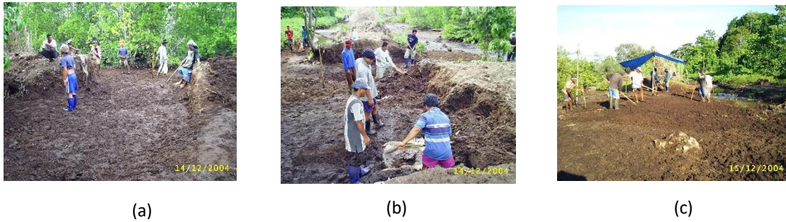
Figure 4. The closing of landward channel at three different points: (a) channel edge connects to the east channel, (b) middle part, (c) near the west channel
