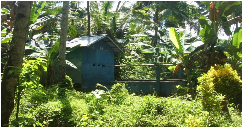
Figure 3. Pumping house and well at the side of village road.
