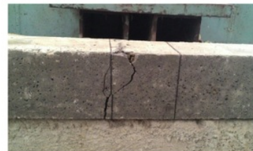
(a). Crack pattern of a beam specimen
