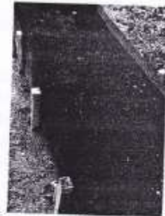
Figure 3. Compacted and Smooth Soil after rainfall (November 17th 2008)
