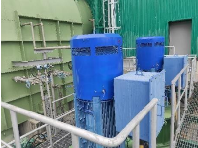
Gambar 2.5 Hot Well Pump
