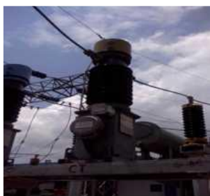
Gambar 1.3 Transformator Arus
