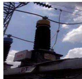
Gambar 1.4 Transformator Tegangan
