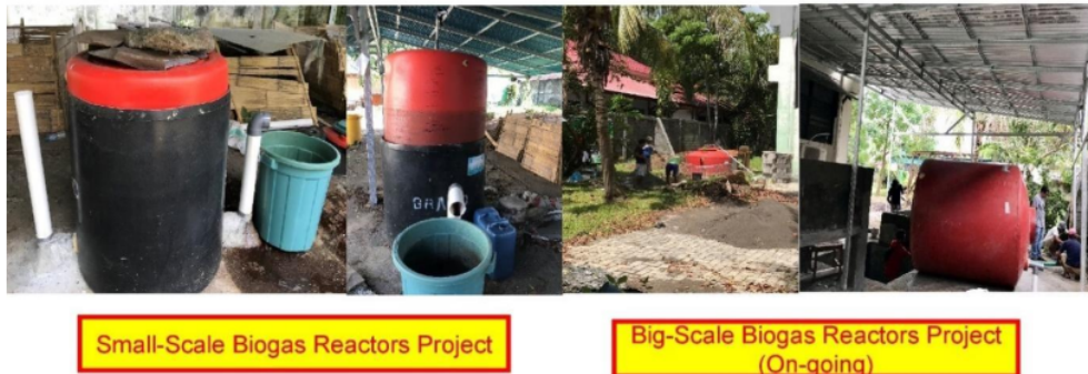
Figure 1. Small-Scale Biogas Reactor Project and Big-Scale Biogas Reactor Project (On-going) at Sam Ratulangi University Manado
