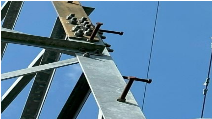
Gambar 11 Step Bolt (T094-T096)
