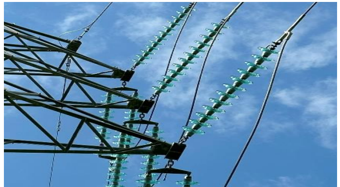
Gambar 7. Piringan Insulator Line 1 (T094-T096)
