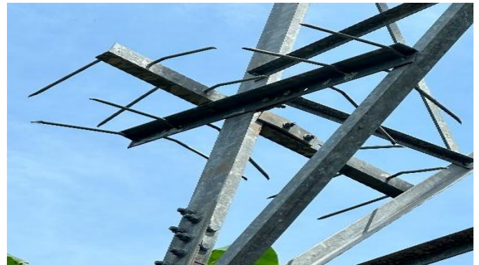
Gambar 12. Anti Climbing Device (T094-T096)
