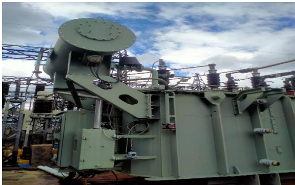
Gambar 2.1 Transformator Daya
