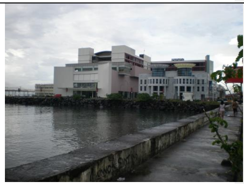
Figure 5. Mall On the Reclamation Area
