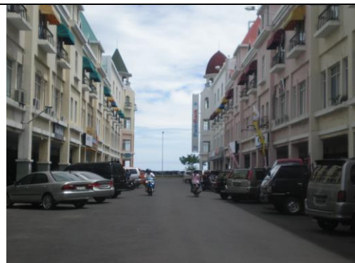
Figure 4. Stores and home office on the reclamation Area
