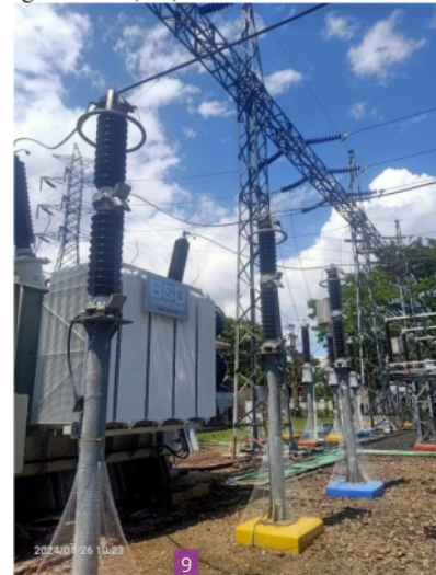
Gambar 2.3 Lightning arrester
